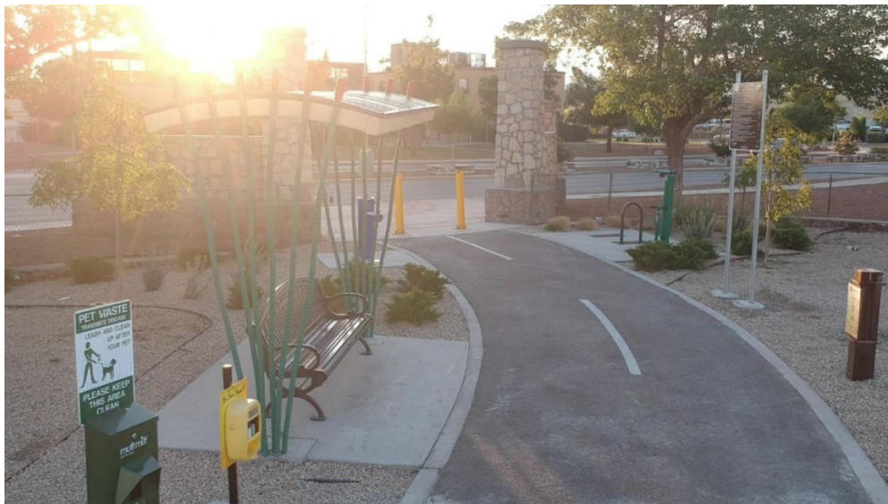
The Playa Drain Trail trailhead at Ascarate Park. The trail includes amenities, landscaping, and lighting.
